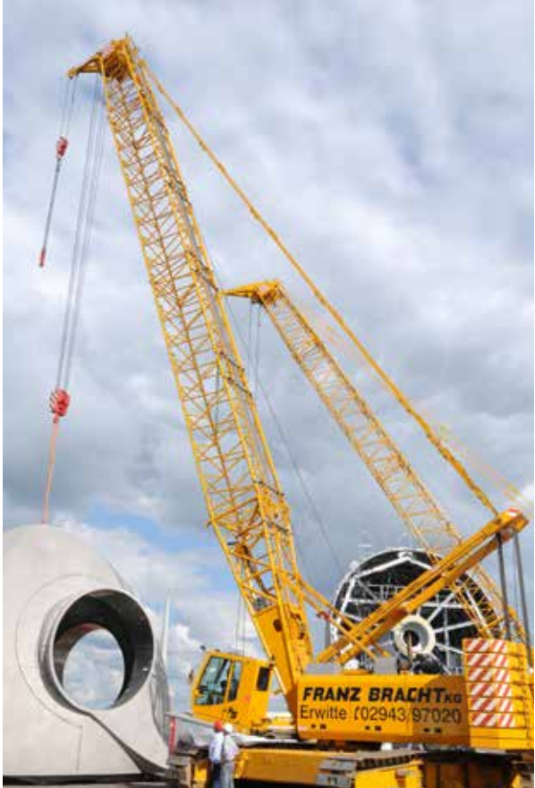
Lattice boom crawler crane deployed in the installation of a wind power station.
